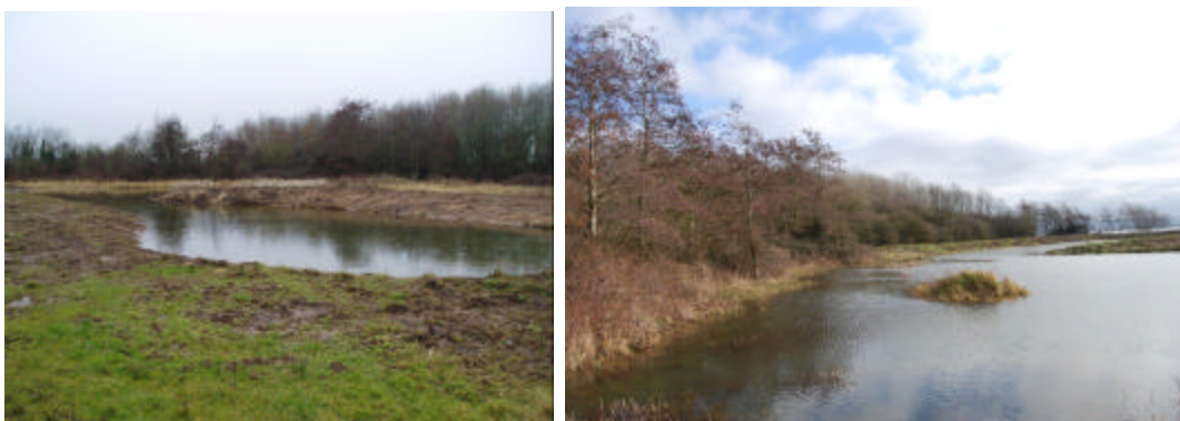
(Above) – recently completed pond restoration works at Poulton Court, Gloucestershire (GWA)
