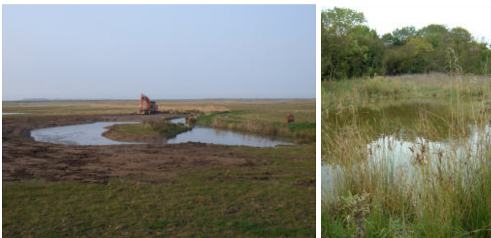
(Above) – Ditch re-profiling at Deepdale Marsh and Bassenhally Pits to provide gently shelving edges for feeding and breeding wildfowl
